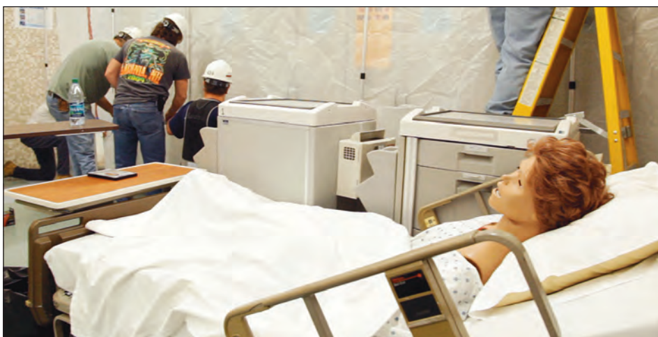
At a recent Best Practices session, Brothers Dave Dann and Bill Thissell of Local 424 (foreground) worked on installing air flow machines while others install soft walls (background and below). The class was held in a nurse's training area at Southeastern Regional Vocational School in Easton to simulate conditions found at an actual worksite.
