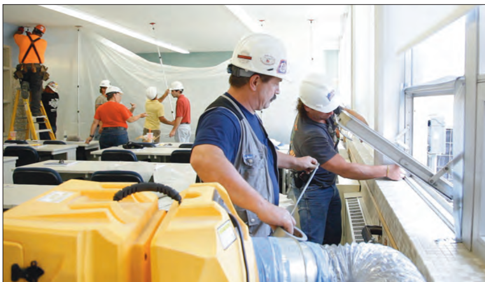
At a recent Best Practices session, Brothers Dave Dann and Bill Thissell of Local 424 (foreground) worked on installing air flow machines while others install soft walls (background and below). The class was held in a nurse's training area at Southeastern Regional Vocational School in Easton to simulate conditions found at an actual worksite.
