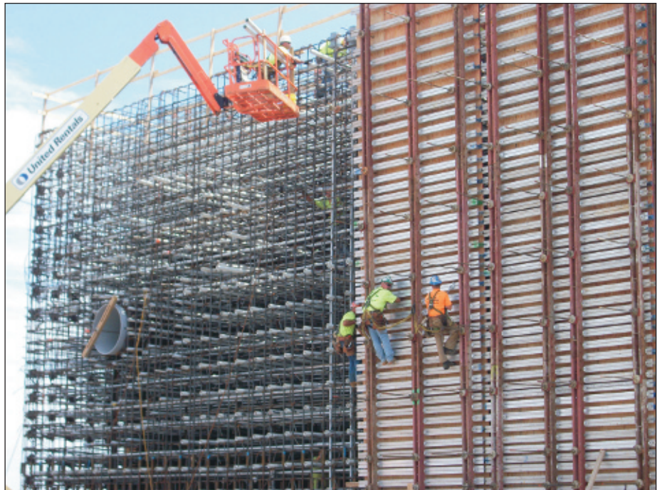
Union Carpenters hang off the side of the forms being used to build a massive structure for testing wind turbine blades up to 90 meters (almost 300 feet) long.
