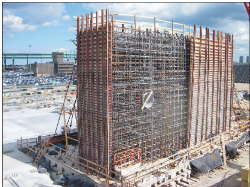
Union Carpenters hang off the side of the forms being used to build a massive structure for testing wind turbine blades up to 90 meters (almost 300 feet) long.
