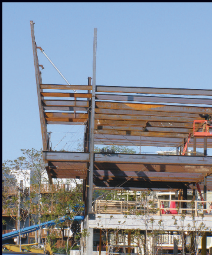
The cantilever was erected in mid-May. The rendering on page 28 shows the LED Display that will be mounted on the face of the cantilever.
