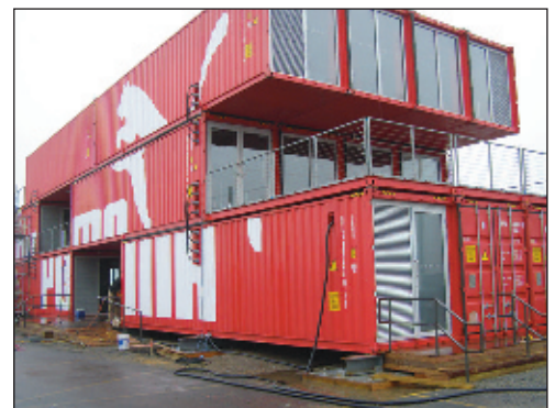
"Puma City" included modular buildings that required assembly and supporting entrances, decks and display to be built.
