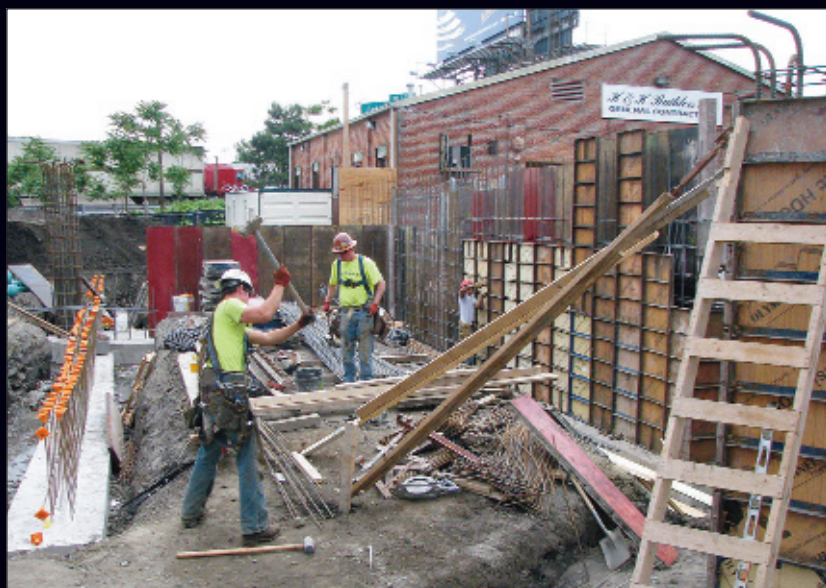
A carpenter works on forms at the parking garage
