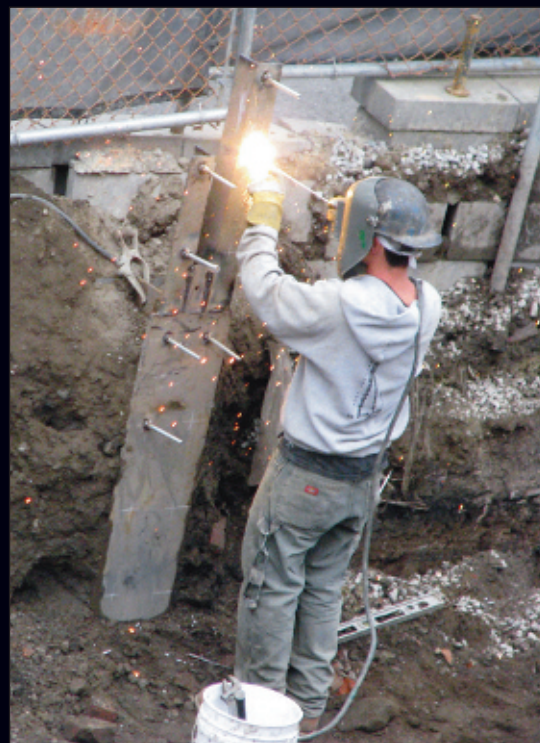
A piledriver works on a soldier pile, used for soil retention.
