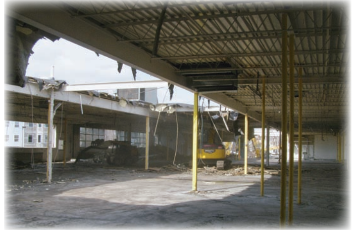
Crews begin taking down the roof from the interior of the second floor
