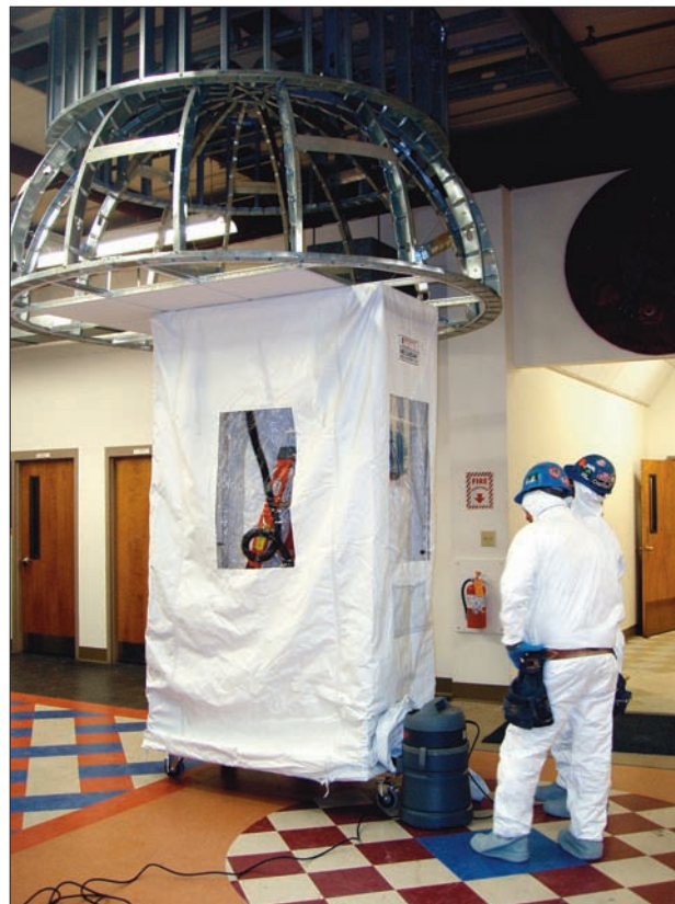
Participants demonstrate how to utilize a "Portable Work Cube" to remove a contaminated ceiling tile from an occupied area.
